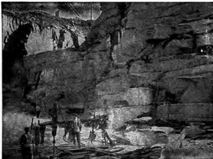
Fig. 25. Rhode Island granite quarry showing the Sullivan "Hy-Speed" Drill and Quarry Bar.
